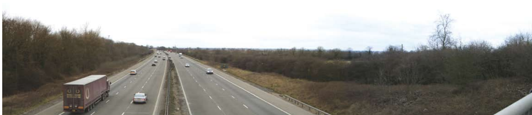
The M1 motorway exerts an influence from the adjacent Character Area
